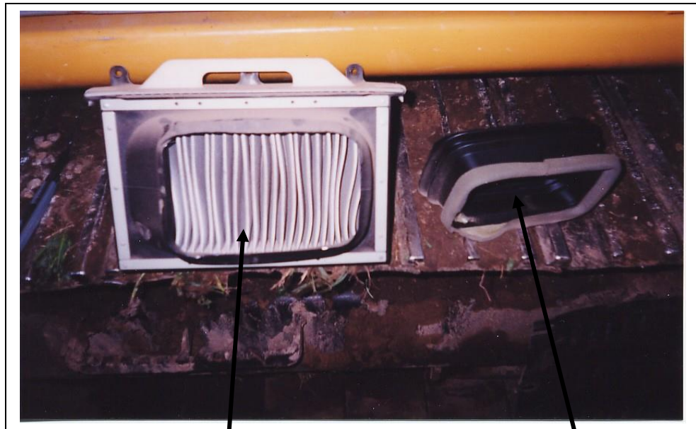
Retain and reinstall once the outside air intake box is mounted to it with self drilling screws and insulation tape.
